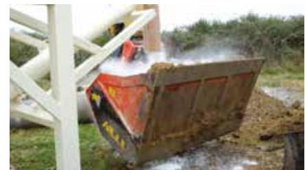
Stabilising soil with lime
