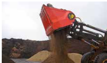
Mixing top soil and sand
