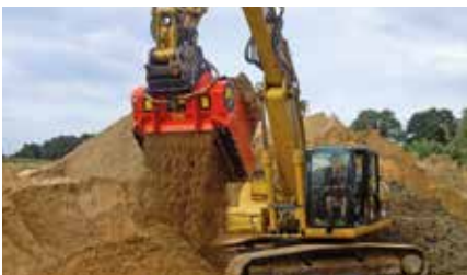
Mixing sand and clay
