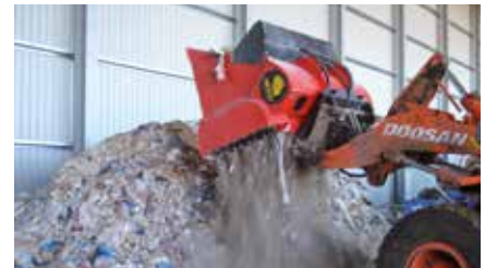
Crushing demolition waste
