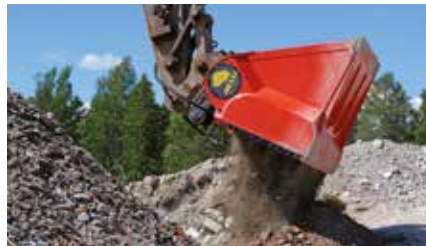
Crushing bricks / black top asphalt
