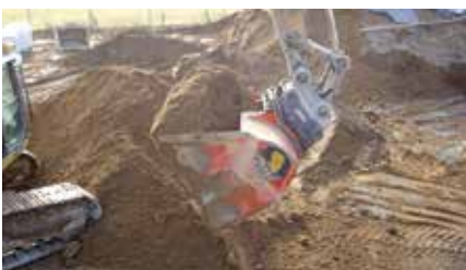
Stabilising foundation layers
