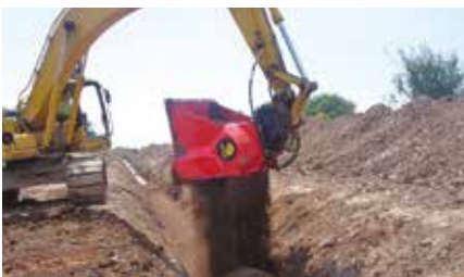
Pipeline padding/back filling
